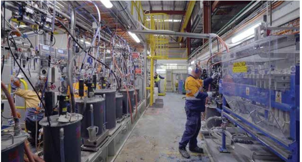
Bundoora Integrated Continuous Chemical Power Plant (BICCPP)
