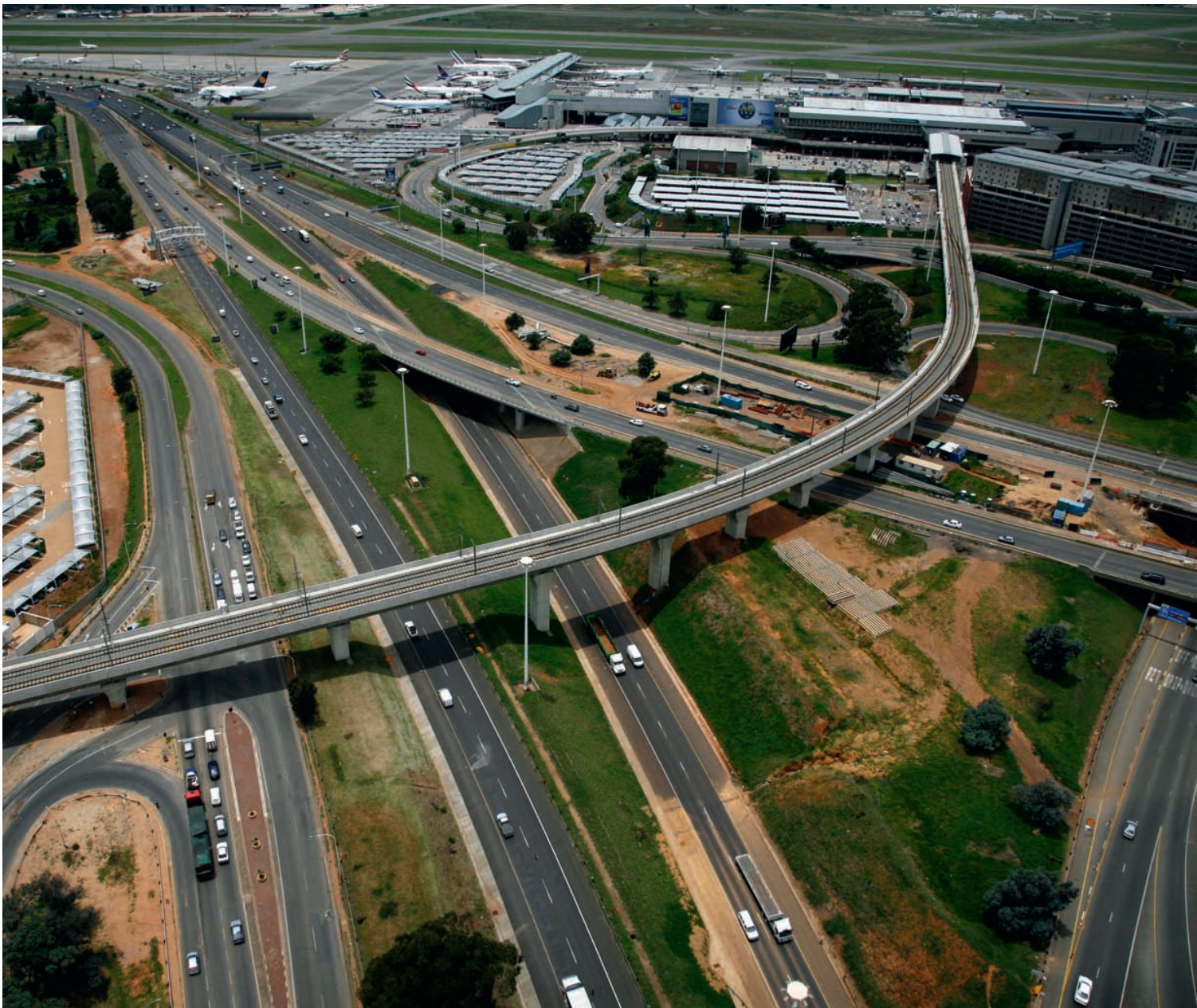
Transport hub at O. R. Tambo International, where Gautrain links up with air terminal and motorways.
