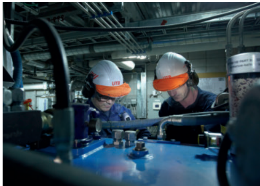
Maintenance workers adjust pump in hydrocarbon section of new plant.
