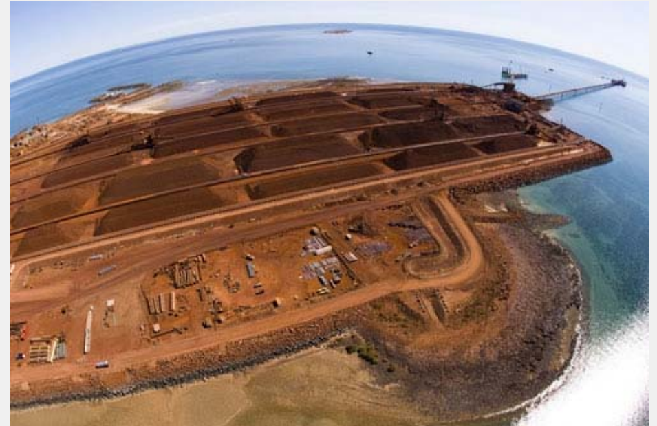
Cape Lambert iron ore port, Australia
