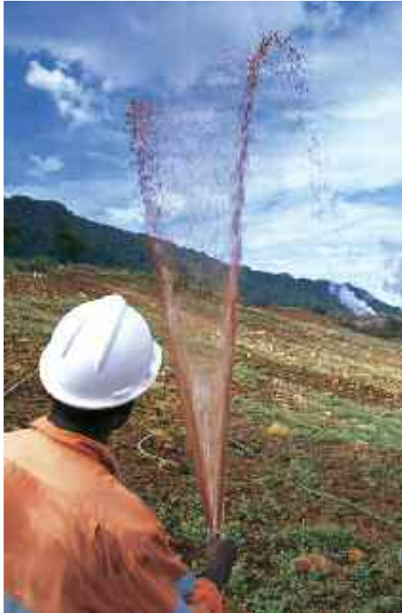
"Hydroseeding" to restore vegetation involves spraying a mixture of seeds, water, fertilisers and mulch onto newly relaid topsoil. Within a month growth will be fully germinated and flourishing.
