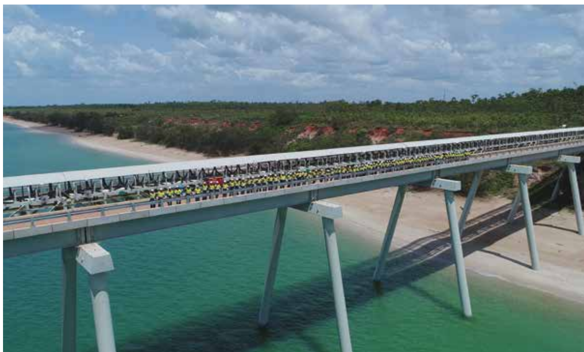
The Chith export facility, comprising a 650-metre access jetty and 350-metre wharf, will serve as a berth for ships while in port.
