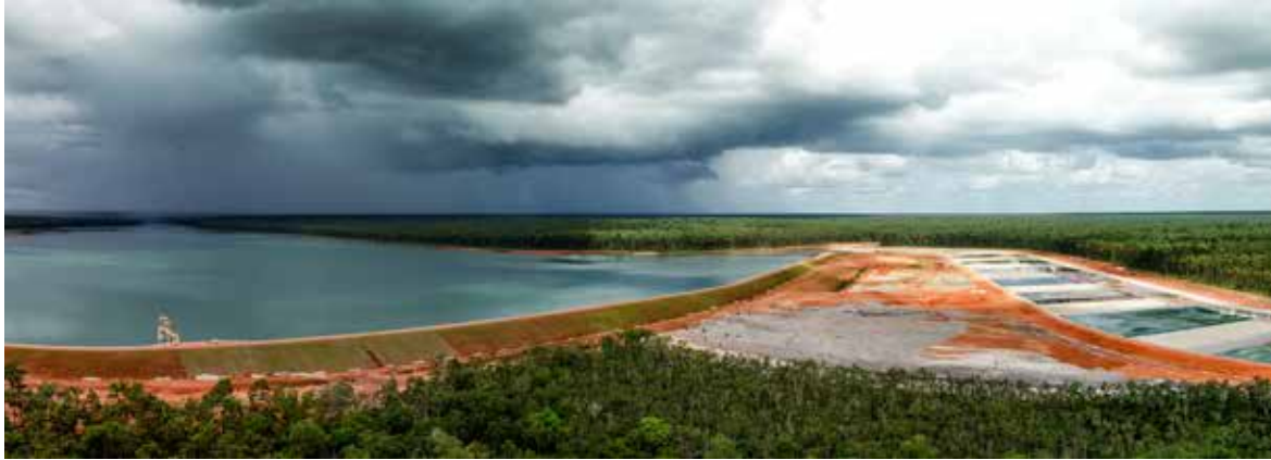
Arraw Dam and spillway with integrated fishway.
