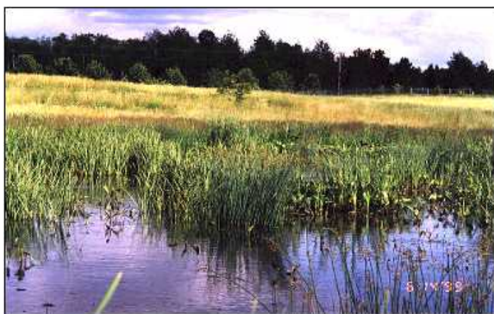
8.5 Acre Constructed Wetland at Flambeau (1999)
