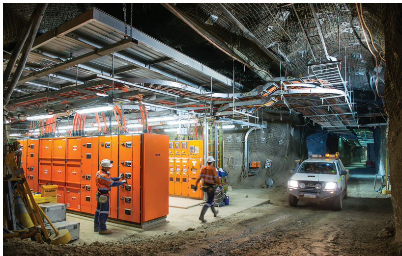
Argyle Diamonds underground mine
