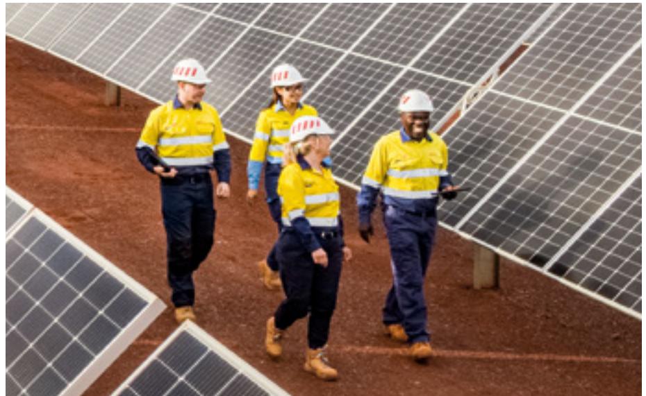
Gudai-Darri solar plant. The Pilbara, Australia
