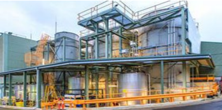
Leaching pilot plant (up to 300 tonnes of ore)
