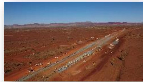
Developing Gudai-Darri mine
